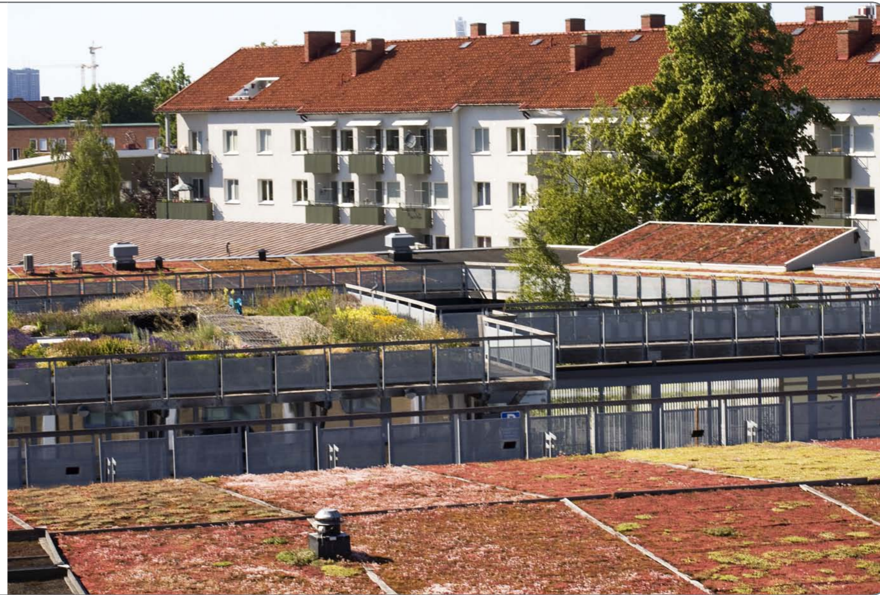
One of many wonderful views of the green roofs.
